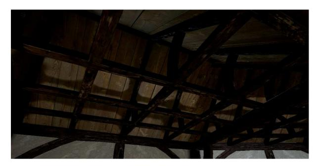
Fig.105: The eaves above the third level gallery showing the queen truss construction overlaid with timber boards
