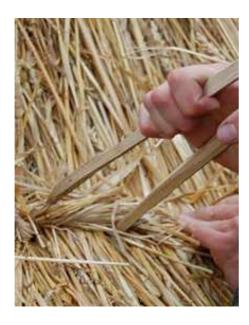
Fig.107 (a): Thatch being stapled with a willow spar
