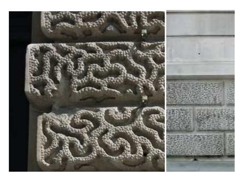
Fig. ?: vermiculated ('worm eaten') ashlar<sup>227</sup>
